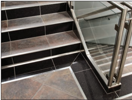
3.3 Schluter®-TREP-E , in stainless steel, installed to provide a durable, slip-resistant stair tread edge and accentuate the design elements of an office building.
